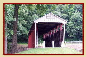
**Year Built:** 1877 Truss type: Howe Length: 68 feet **Builder:** J.S. Fleming Crooked Creek Stream:
