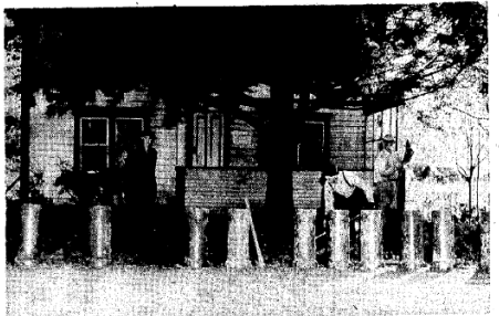
Great Conrad, 71, descendant of one of the founders of Smithsburg, looks on regretfully as borough employees Joshua Lewis and G. L. Welsh remove the sewer pipes along Church street in preparation for the complete evacuation of one-half of the old farm town. The house, like nearly all those still standing in this section of town, is marked with the "No Trespassing" sign which indicates that it has already become U. S. government property.
